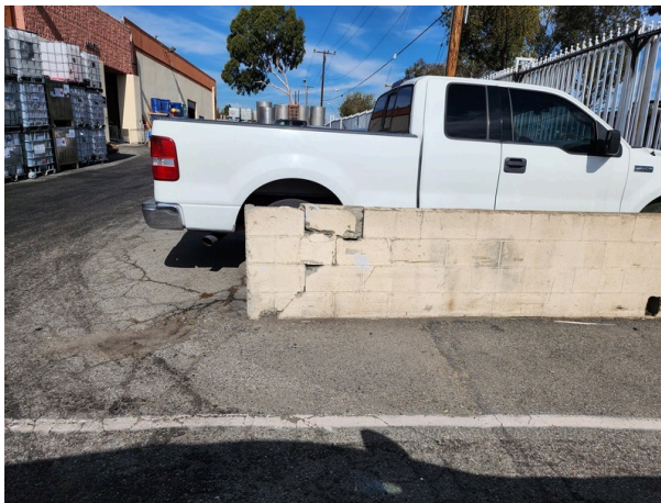
Damaged CMU wall at entrance.
