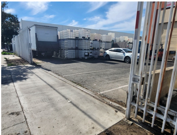
Concrete approach apron at in use entrance.
