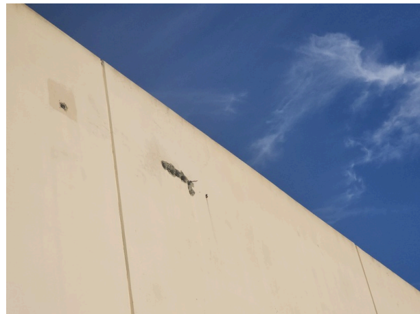
Holes in parapet wall.
