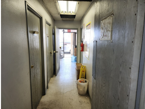
Missing ceiling tiles and damaged/stained flooring.
