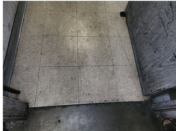
Damaged and stained vinyl flooring and trim.
