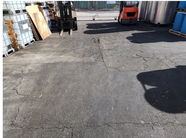
Additional asphalt with concrete patching.
