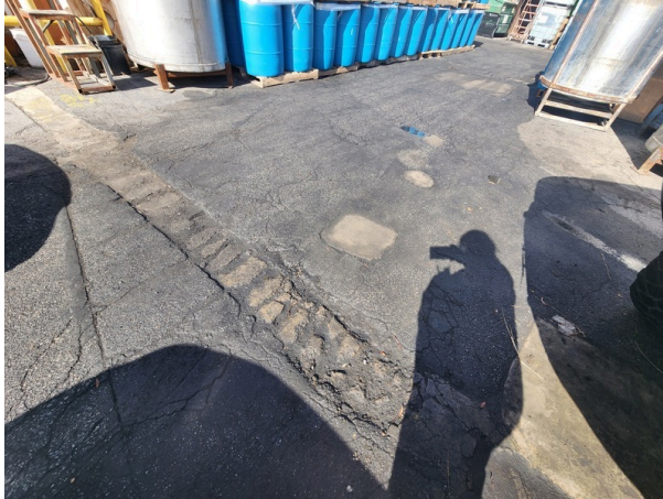
Degraded asphalt pavement.
