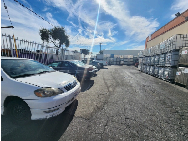
Extensive cracking of asphalt paving and faded parking stall striping.
