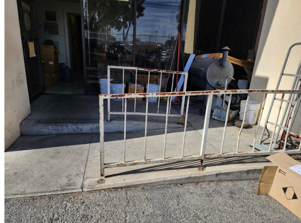
Railing at entrance which is damaged and rusted.
