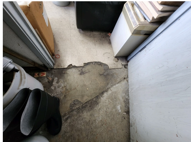
Laboratory flooring is damaged.
