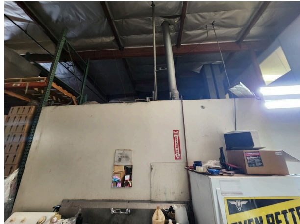
No longer in use ductwork.
