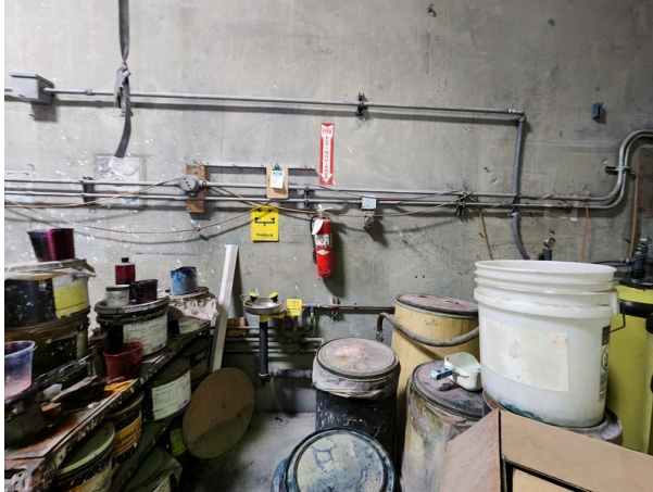
Water lines to eye wash station in mixing area.
