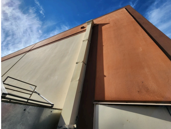
Downspouts and overflow scuppers.
