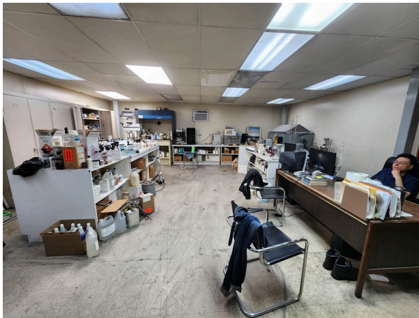
Laboratory finishes. Vinyl tile flooring is damaged and ceiling tiles are aging out.
