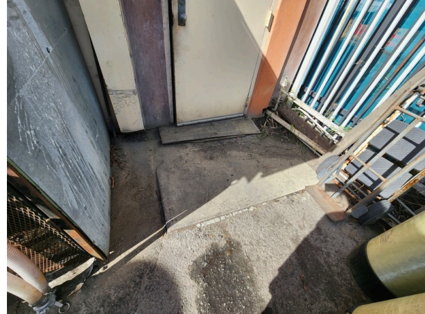
View of northeast elevation of building showing depression directing storm water toward building foundation.
