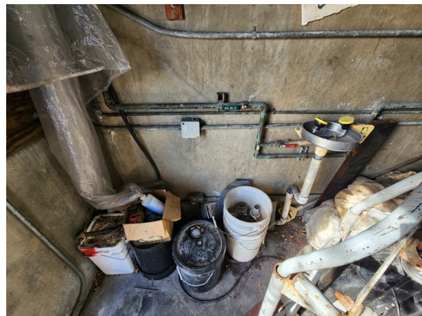
Copper water lines near eye-wash station are corroded.
