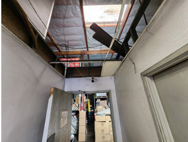
Corridor outside offices: missing ceiling tiles and damaged wooden door.
