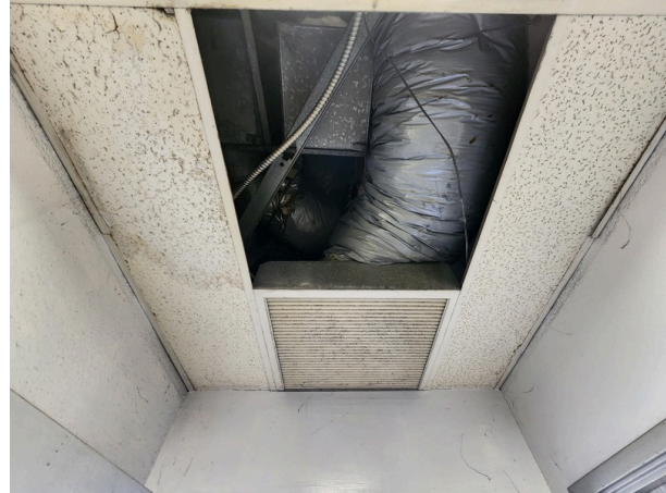
Office hallway: additional missing and aged-out ceiling tiles.
