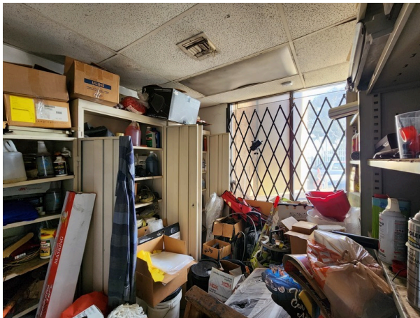
Office area: ceiling tiles are aging out and ceiling vent needs to be replaced.
