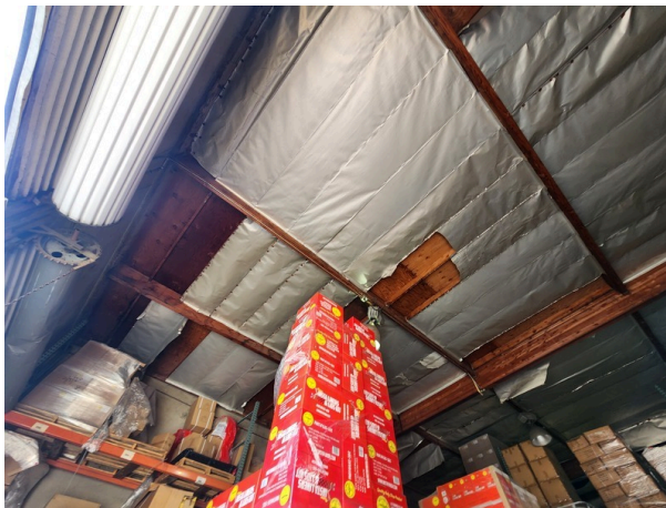
Tear in ceiling insulation shows roof decking.
