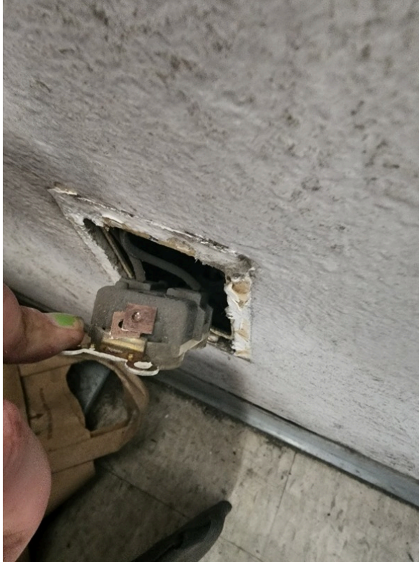
Outlet in office was not secured to wall.
