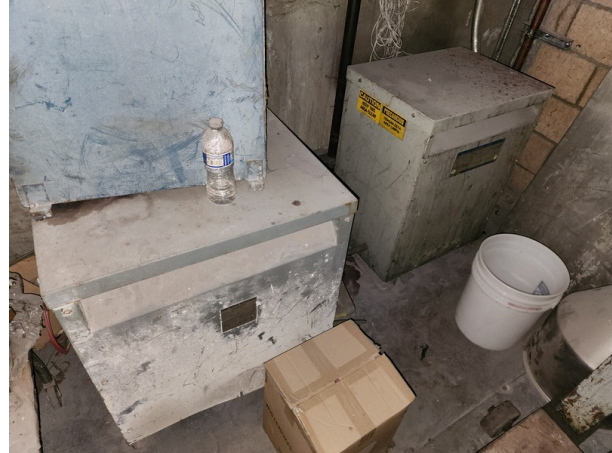
Dry-type interior transformers near main switch.
