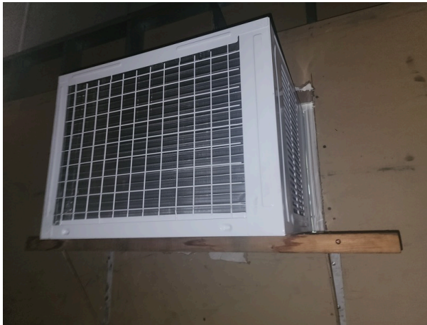
Office through-wall air conditioner.
