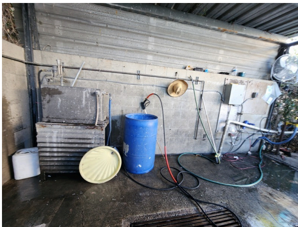
Copper water lines in exterior wash area.
