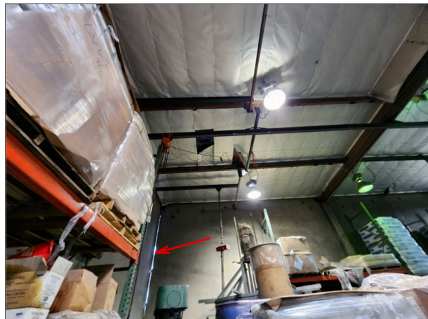
Daylight visible between walls.
