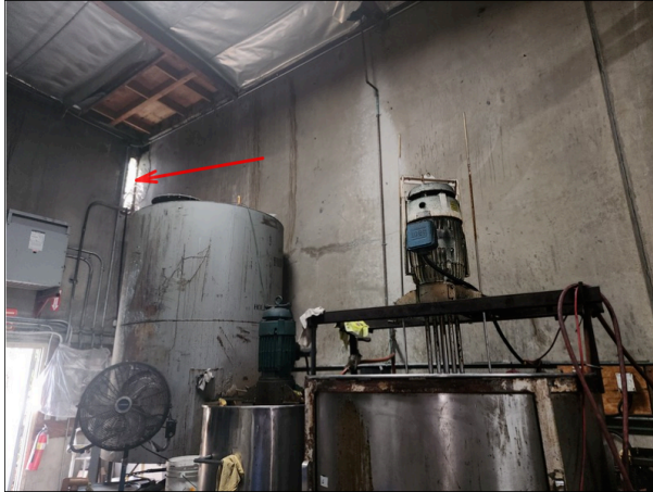
Daylight visible at junction between two walls.
