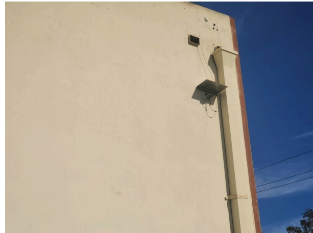
Parapet drain and scupper with missing downspout.
