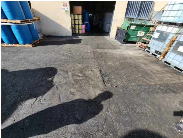
View of asphalt paving with concrete patching.
