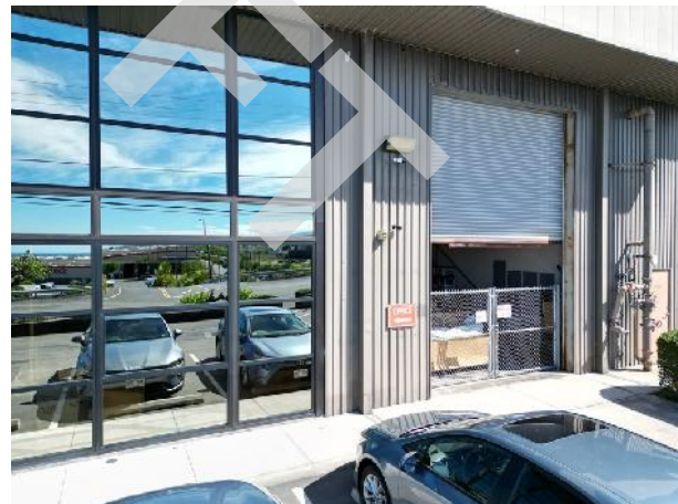
Glass at front, steel siding and roll up door
