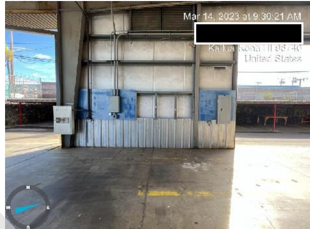
Floor staining beneath insulation damage
