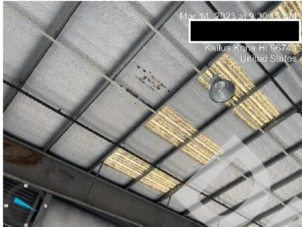
Damaged insulation
