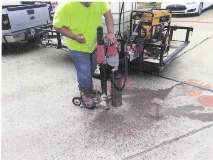
Photograph 2, view facing Southeast: Coring asphalt preparing to advance B-1.
