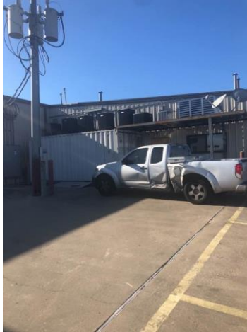
Eastern exterior wall: pole-mounted transformers.
