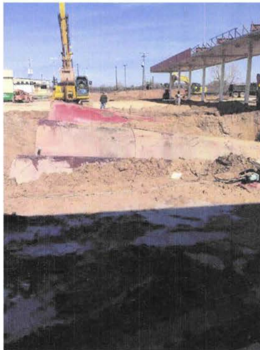
Photograph 4: Facing North, Excavation and removal of three diesel tanks (Diesel Island)
