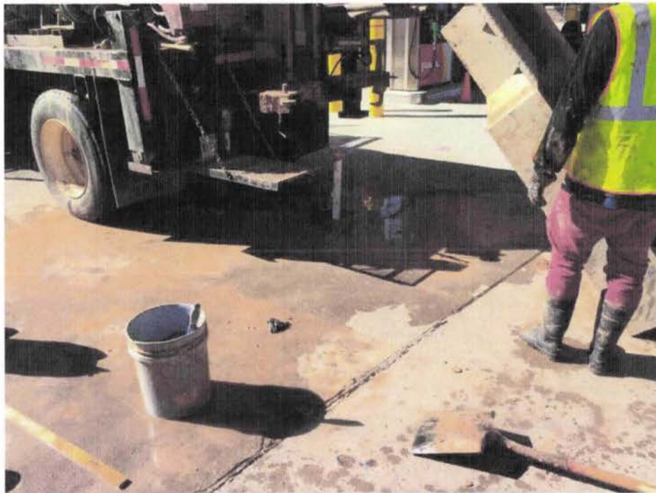
Photograph 8, view facing Northwest: Setting PVC casing to complete boring B-3 as monitoring well MW-3.
