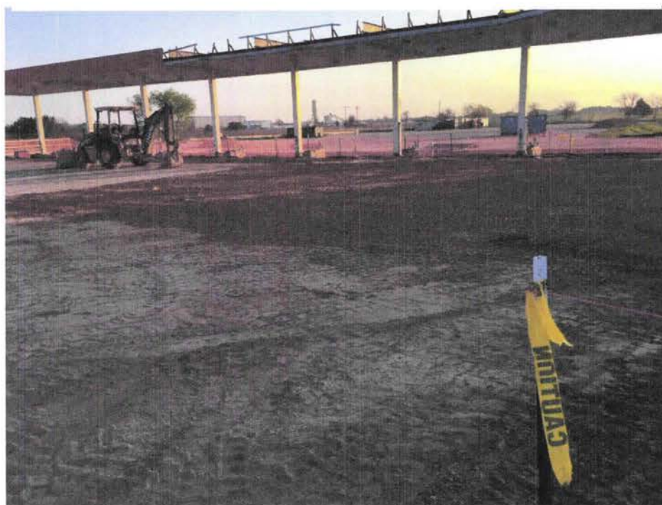
Photograph 6: Facing Northeast, Tank hold backfilled to grade (Diesel Island)
