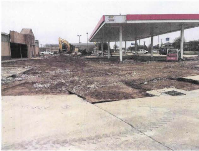
Photograph 3: Facing West, Tank removal activities continue (Commercial Island)
