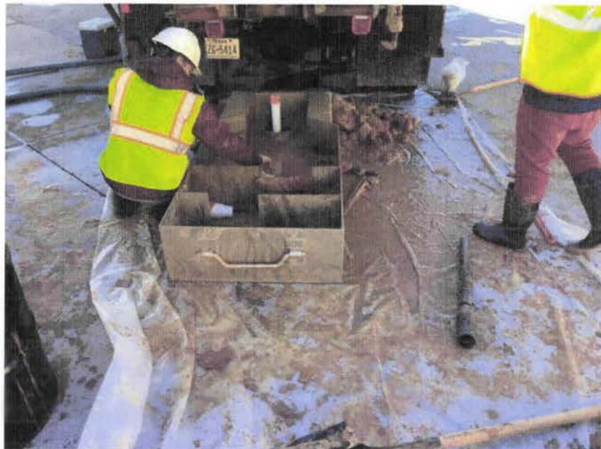
Photograph 6, view facing Southeast: Setting PVC casing to complete boring B-2 as monitoring well MW-2.
