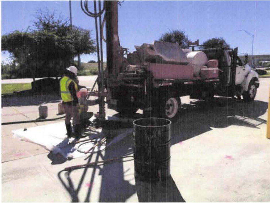
Photograph 7, view facing South: Advancing boring B-3.
