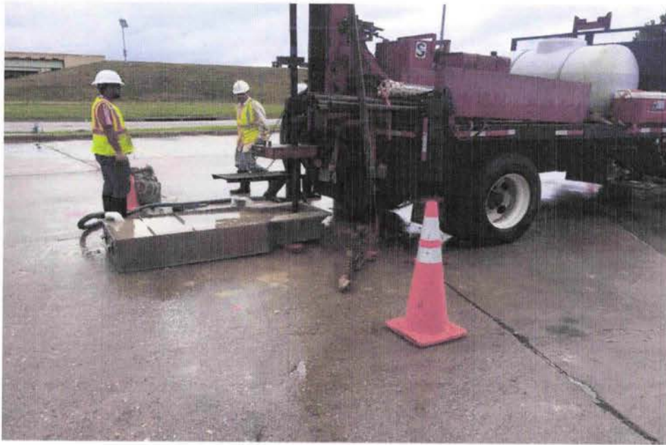
Photograph 3, view facing Southwest: Advancing boring B-1.
