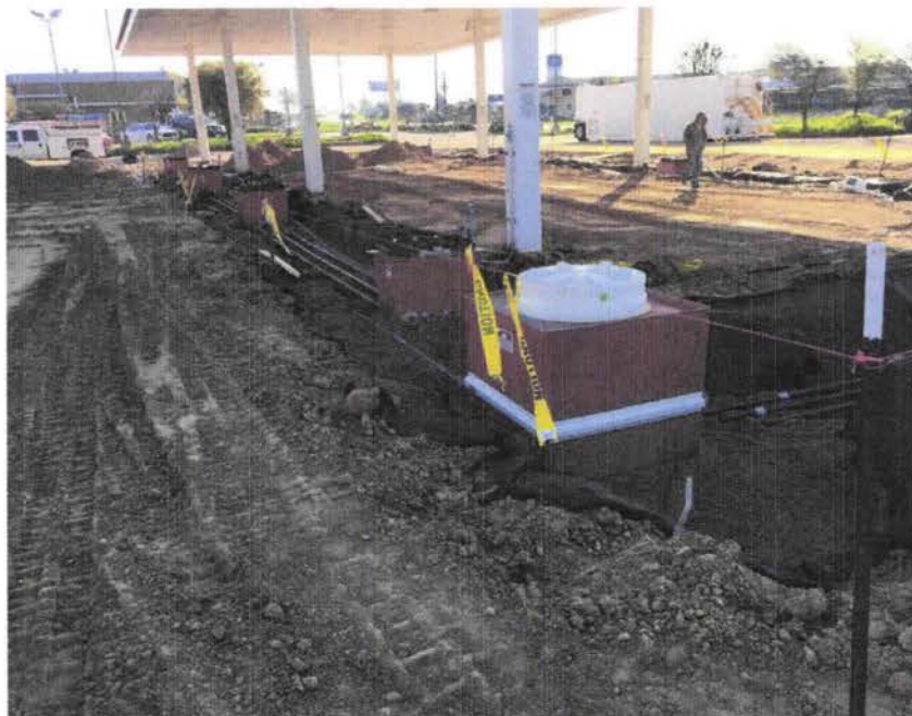
Photograph 5: Facing East, New sumps and product lines placed in trenches (Commercial Island)
